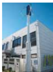
Vertical wind power generation system, which is quieter than the propeller type
