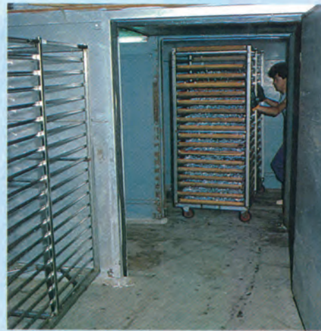
Entering the drying room. The dryer features two modes: a cool blower (22-23°C for 17-18 hours) and a hot blower (40°C for 15-16 hours).
