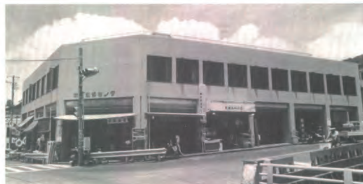
Kozushima Fisheries Cooperative. The 2nd floor holds the Cooperative's offices, and the first floor is store space for rent.
