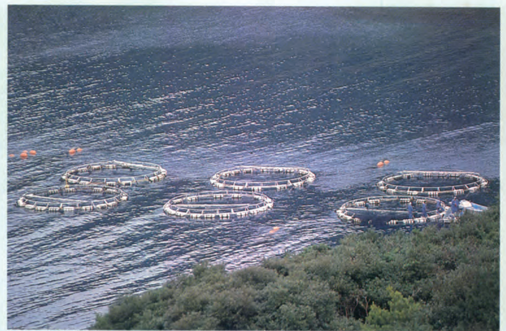
In recent years we have seen the appearance of circular net cages utilizing galvanized steel pipes of 50mm diameter and held up by steel floats with a flotation capacity of 200~250kg.
