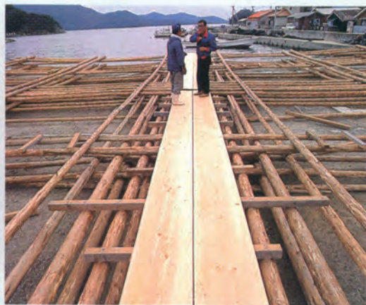
The raft construction of the culture facility diagramed in FIG. 8-2. Down the center is a board walkway that serves as an access for feed distribution and other jobs.
