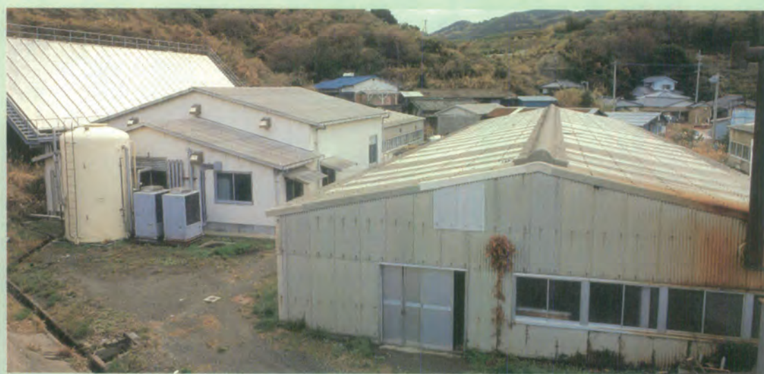
A seed production facility (Nagasaki Prefectural Culture Research Center). In the lefthand building are holding tanks for parent fish and hatching facilities. In the righthand building are tanks for the primary rearing stage of fry. The panel on the left gathers solar energy to heat the water in the parent holding tanks.
