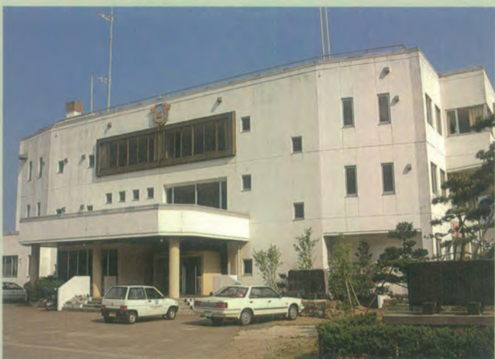
The office building of the Hiranai-cho Fisheries Cooperative Association
